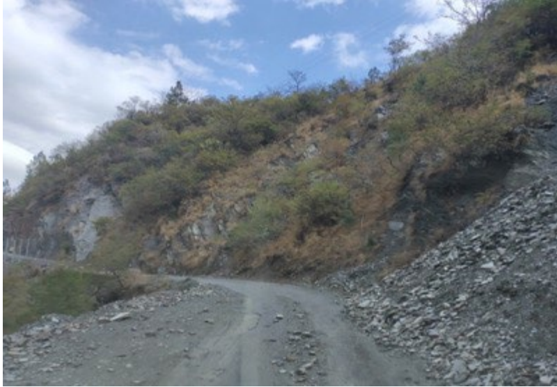
Landslide prone areas in tourism road
