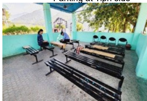
Waiting Area at Madan Negi Station
