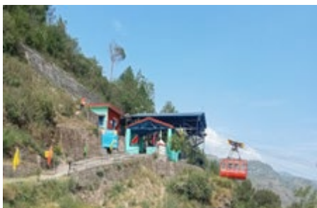
Tipri Ropeway Station
